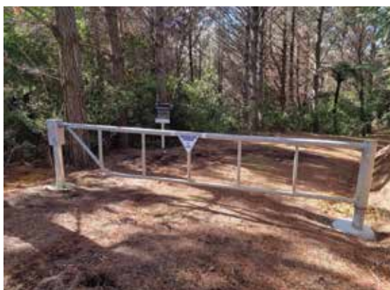
Above left: New Security gate installation. Avoca Forest, Northland
